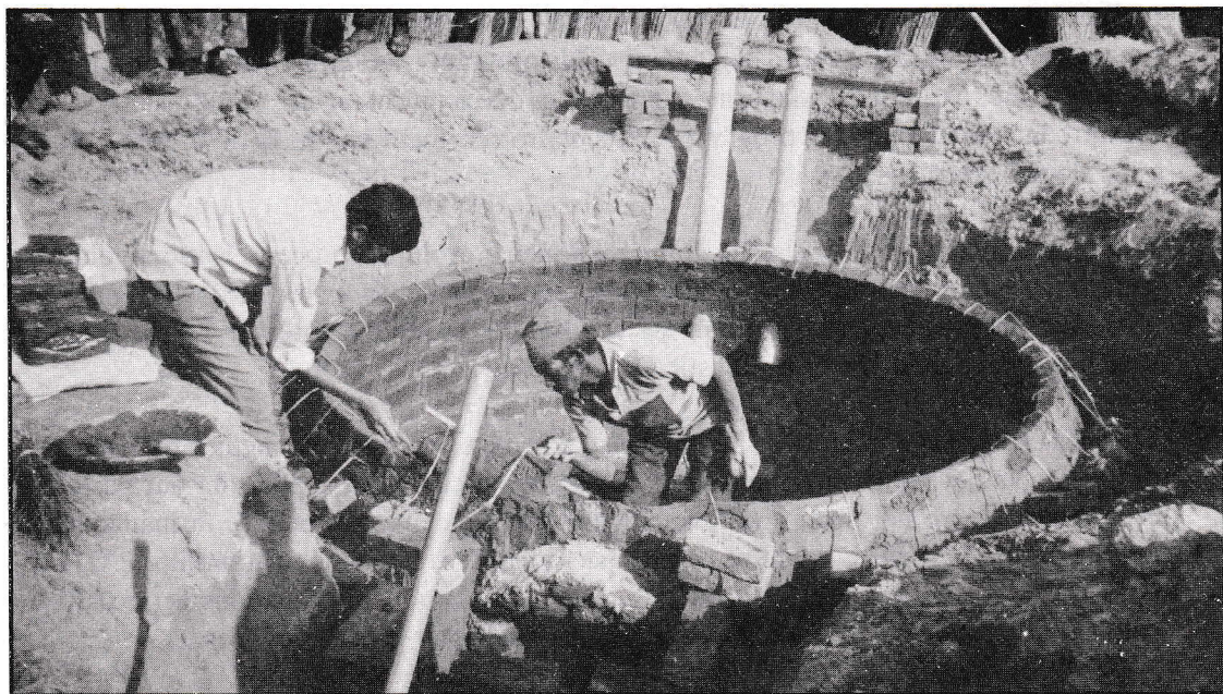
A Biogas Plant being constructed
